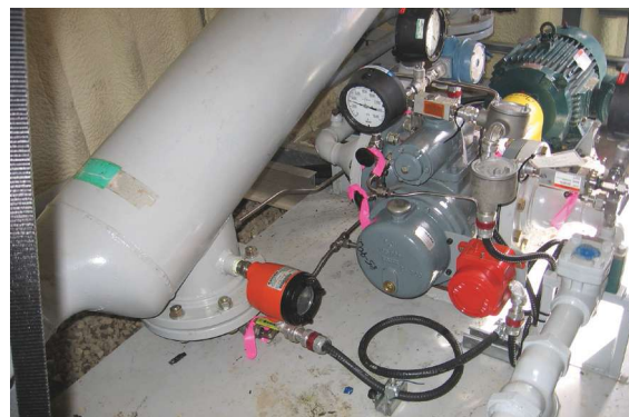
The Leistritz MAGU system, shown in operation, keeps the annulus gas pressure down and maintains the tubing level. (Photo courtesy of Leistritz Advanced Technologies Corp.)
