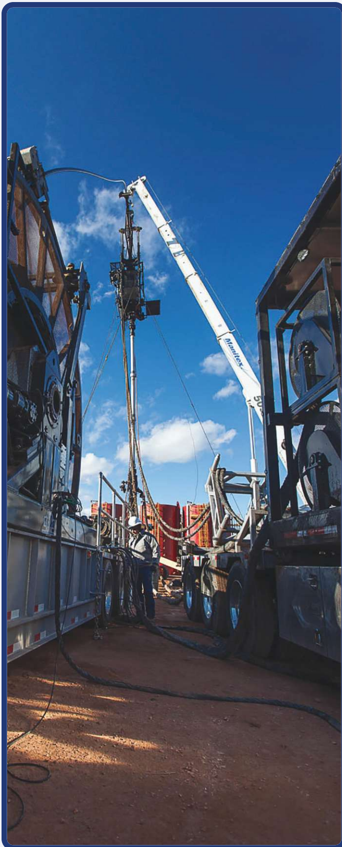
C&J's AR12 is a coiled tubing unit on location in North Dakota. (Image courtesy of C&J Energy Services Inc.)
