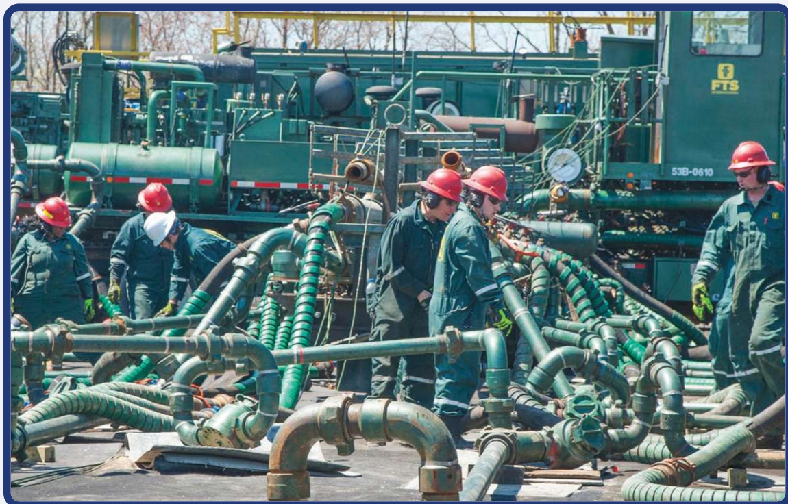
FTS employees rig up on location at a well site. (Image courtesy of FTS International)
