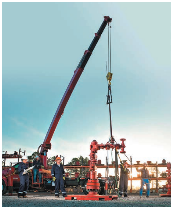
A surface valve installation of an IS-A backpressure valve at the TechnipFMC training facility took place in Tomball, Texas. (Photo courtesy of TechnipFMC)
