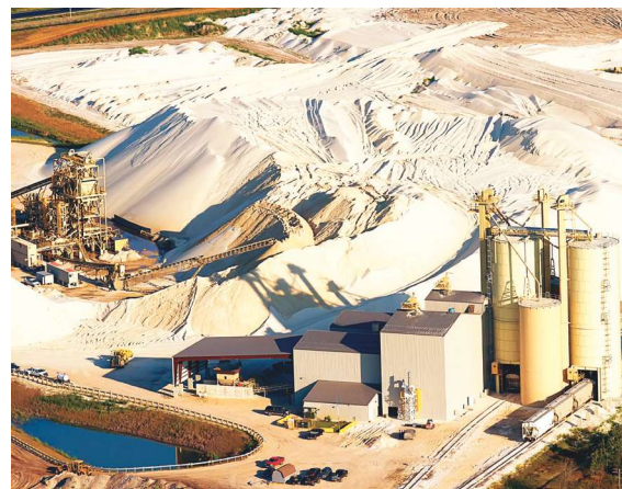
The Hi-Crush processing facility near Wyeville, Wisconsin, can produce 1.85 million tons/year of 20/100 fracture sand. (Photo courtesy of Hi-Crush)
