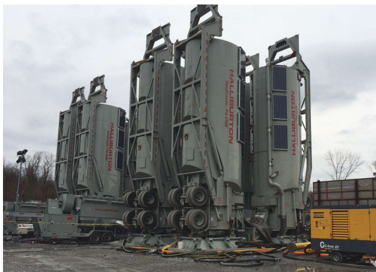
Halliburton’s SandCastle PS2500 proppant storage systems are on location at CONSOL Energy’s Pittsburgh International Airport project. (Photo courtesy of Halliburton)
