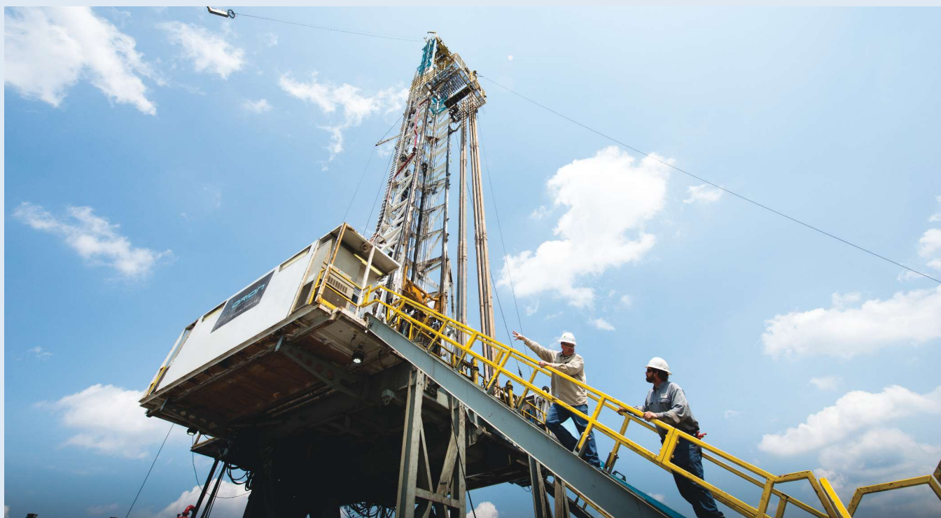
Statoil's Marcellus operations in Wetzel County, W.Va., make up part of the company's 512,000 net acres targeting the play. (Photo by Ole Jørgen Bratland, courtesy of Statoil ASA)
