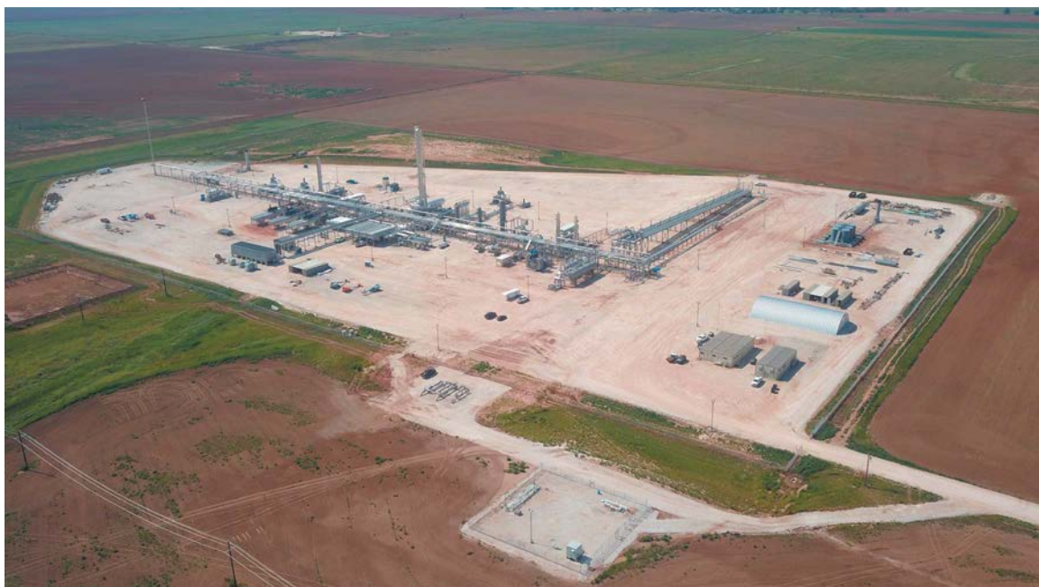
Canyon Midstream’s Redcliff gas-gathering, treating and processing project in the Stack play has been in service since April 2018. The system comprises a 200 MMcf/d cryogenic plant in Woodward County, 155 miles of gathering line, and five field compression stations in Woodward, Dewey, Blainem and Canadian counties. The Redcliff system delivers residue gas to ANR and Southern Star, and NGLs to ONEOK. (Photo courtesy of Kayne Anderson Energy Funds)
