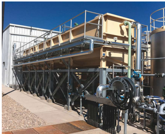
A custom-designed Hydrasep handles both oils heavier than water and lighter than water. (Photo courtesy of Hydrasep)
