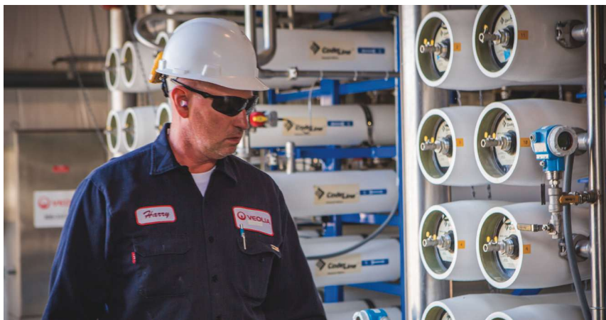
Veolia’s OPUS II technology is a membrane-based process that generates effluent suitable for discharge to surface water or reuse for crop irrigation—a significant benefit in water-strapped regions. (Photo courtesy of Veolia Water Technologies)
