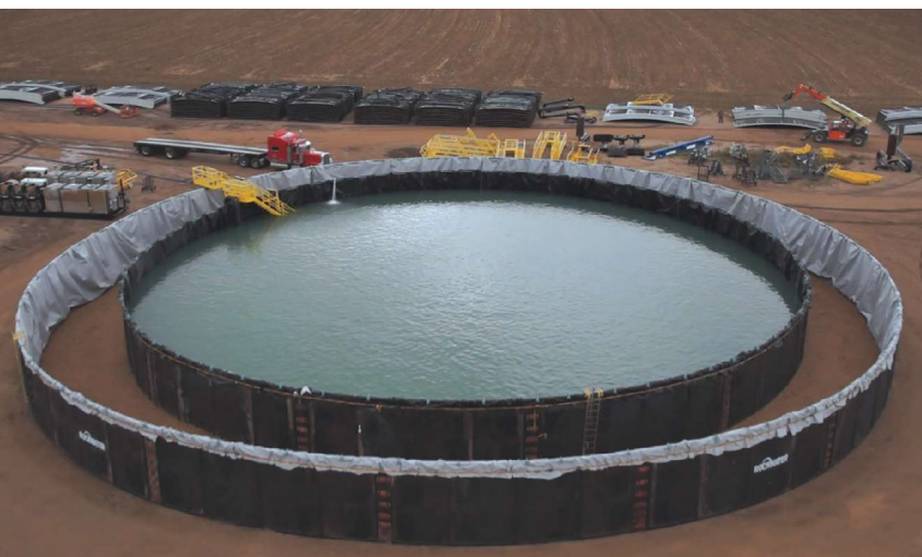
Rockwater aboveground storage tanks are approved to store produced water in six states. Pictured here is a nested tank configuration to provide secondary containment. (Photo courtesy of Rockwater Energy Solutions)
