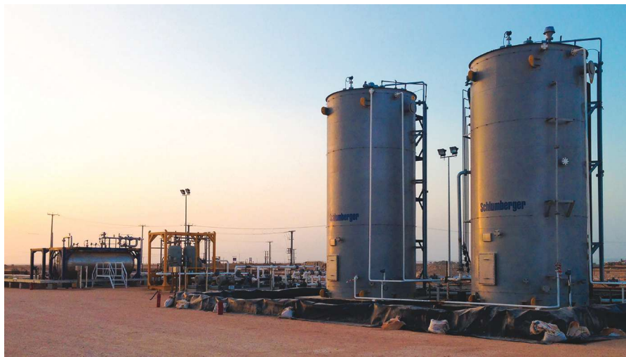
The EPCON DUAL compact flotation unit enables bulk oil removal through polishing of water in half the footprint of conventional technologies. (Photo courtesy of Schlumberger)
