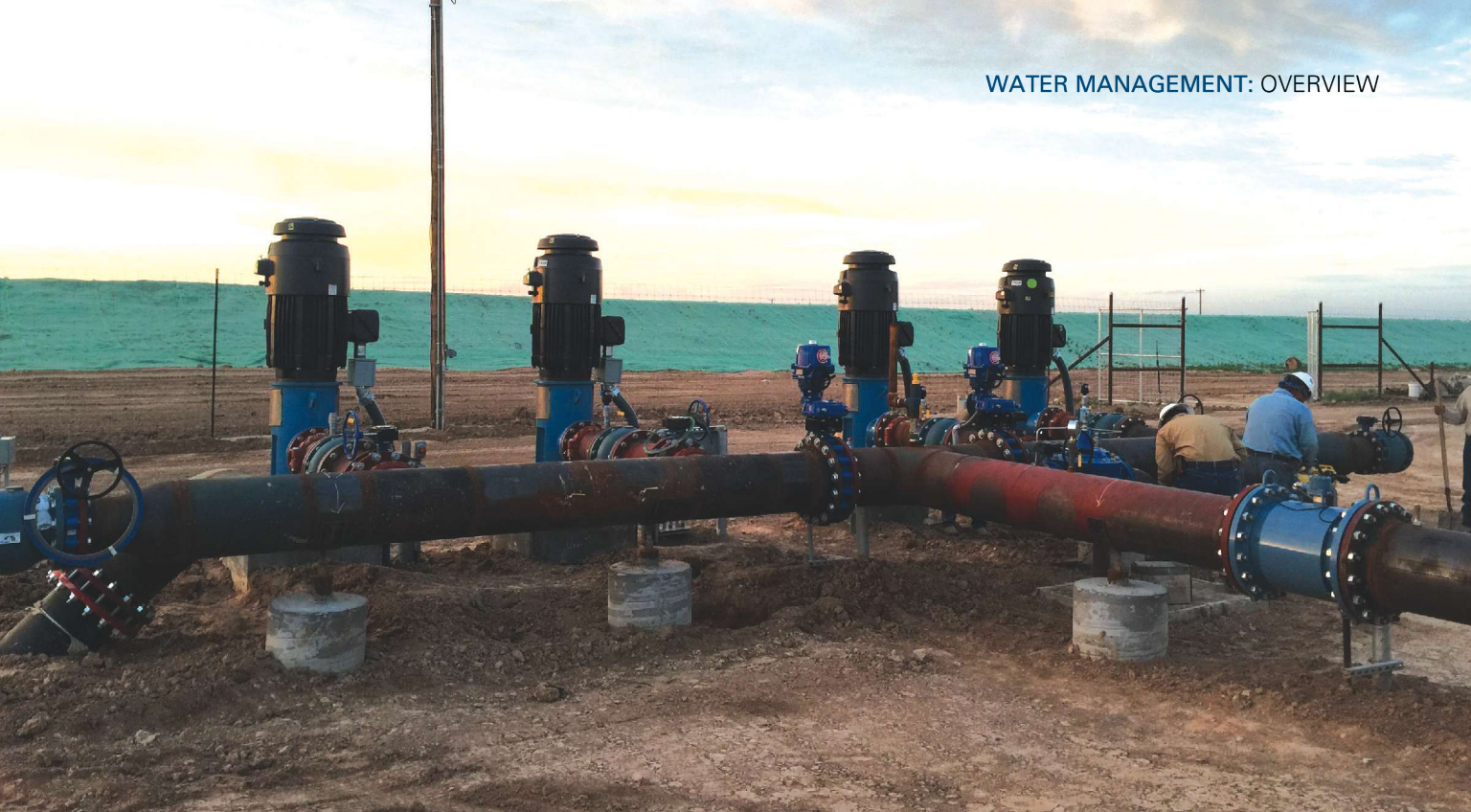
Layne Christensen's pump station operates four pumps running at 125 hp each and can pump more than 175,000 bbl/d of water through the company's Hermosa pipeline. (Photo courtesy of Layne Christensen)
