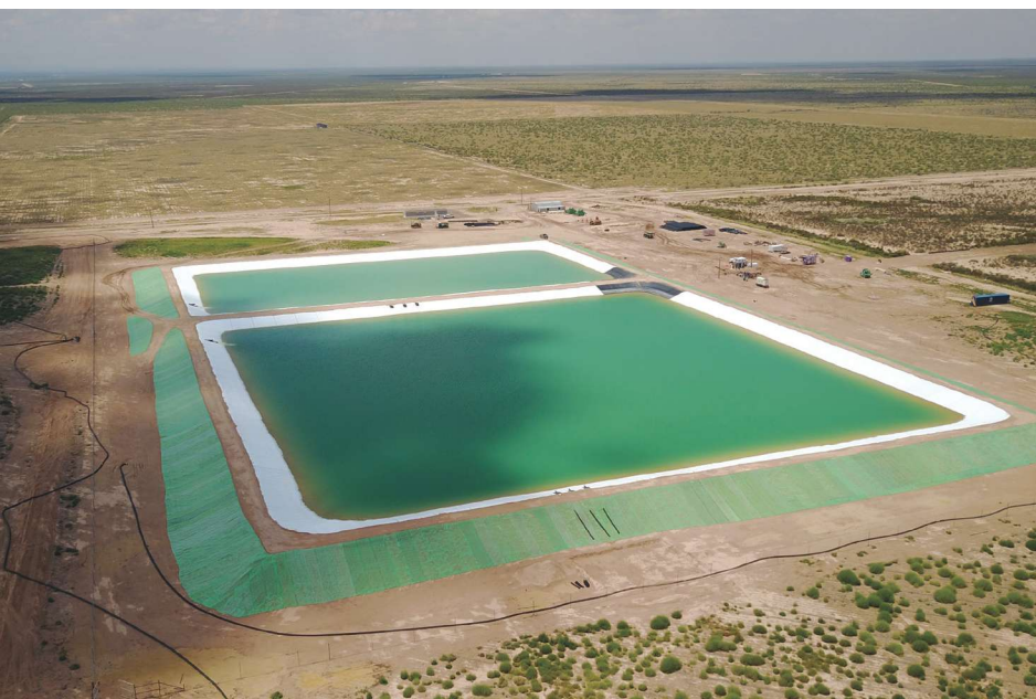
Layne Christensen operates two freshwater storage ponds just outside Pecos County in the Permian Basin, one holding 500,000 bbl and the other holding 250,000 bbl of water. (Photo courtesy of Layne Christensen)
