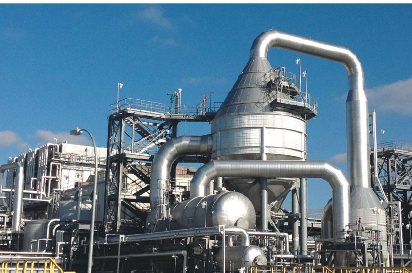
The modular MBD is designed to shorten project schedules and save installation costs. (Photo courtesy of Veolia Water Technologies)
