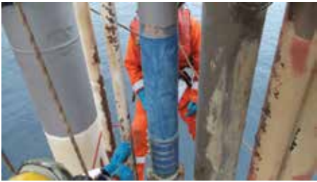
Trained installers using rope access apply filling material to the defect and use adhesive to secure the repair sleeves on an asset in the North Sea. (Photo courtesy of Clock Spring Co. Inc.)
